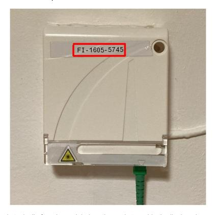
The OCP identifier is typically found on a label on the socket, and is the line's unique and permanent ID. The format may vary, e.g. ZM-1234-1234. On the above photo, the OCP identifier is circled in red.
